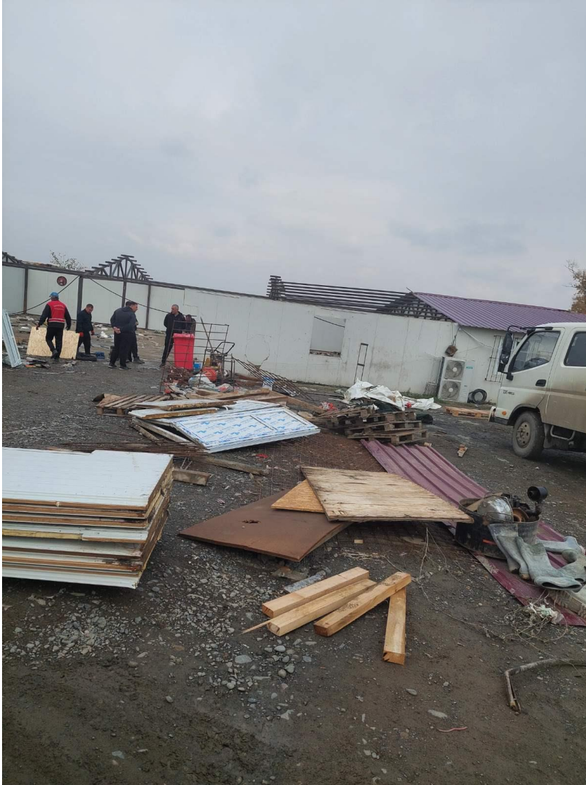
Dismantling of Anaga workshop buildings
